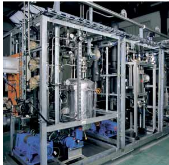
Stirred reactor test plant
