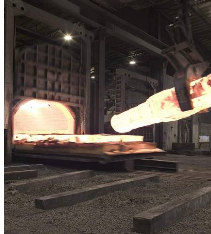
Car bottom furnace at SCANA Steel, all equipped with flameless oxyfuel
