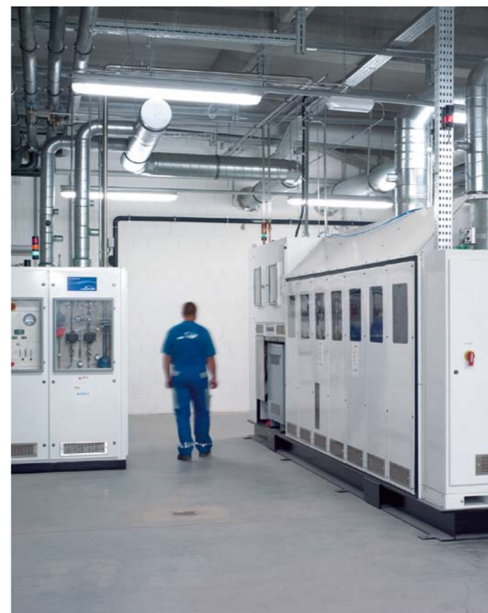
On-site fluorine generator for chamber cleaning
